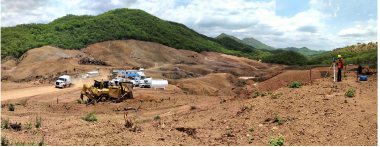
Figure 1: Heap Leach Pad Construction at Santana
