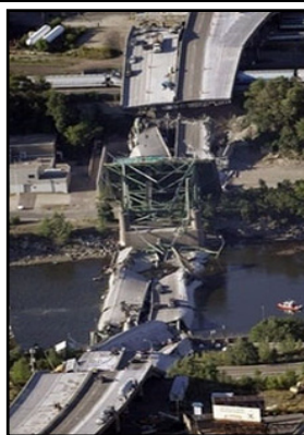
Figure 3 MINNEAPOLIS BRIDGE COLLAPSE
