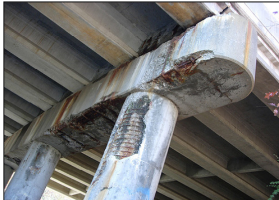
CONCRETE SUPPORTS CORRODED DOWN TO THE STEEL REINFORCEMENTS
