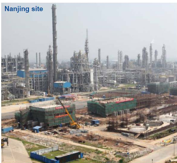
Figure 79: Nanjing site expansion currently underway
