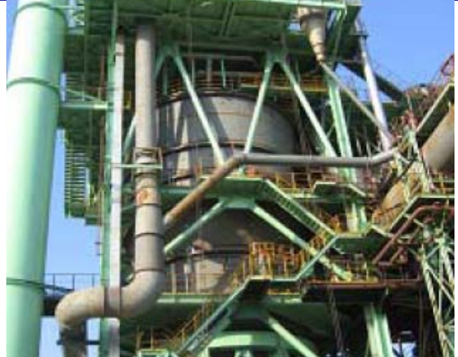
Figure 60: CDQ (Code Dry Quenching) waste heat boiler
