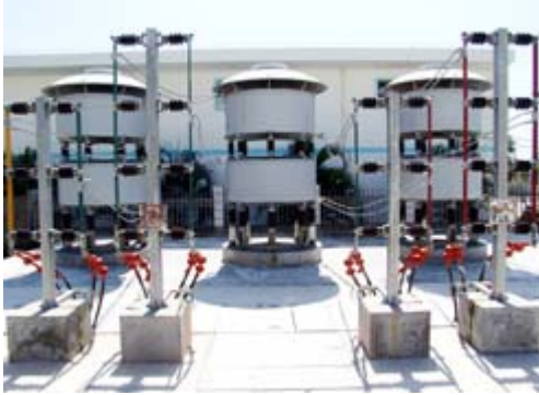
Figure 108: Compensation equipment
