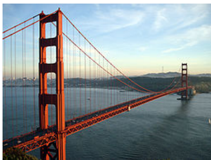
Golden Gate Bridge, San Francisco.
