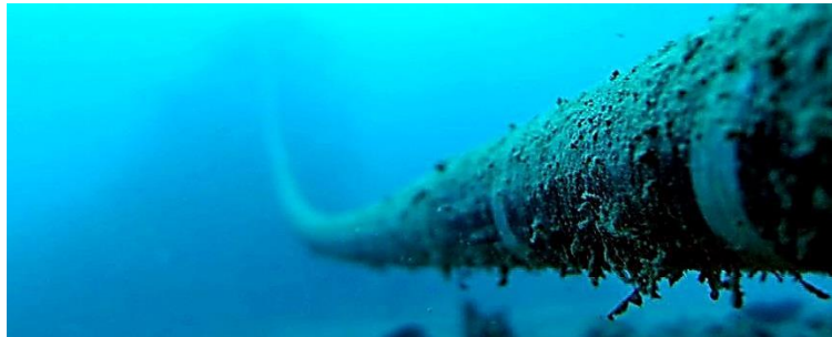
Fig. 37 – Vegetation colonization of a submarine cable (Source: orange.com )
