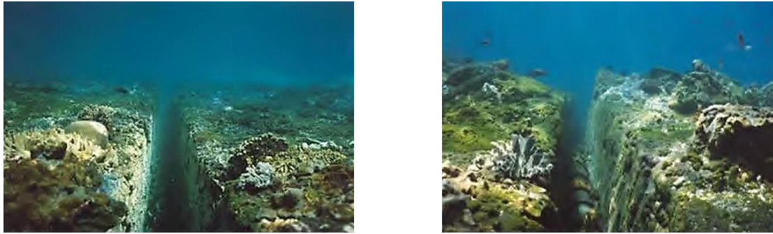
Fig. 31 – The trench of a submarine power cable
