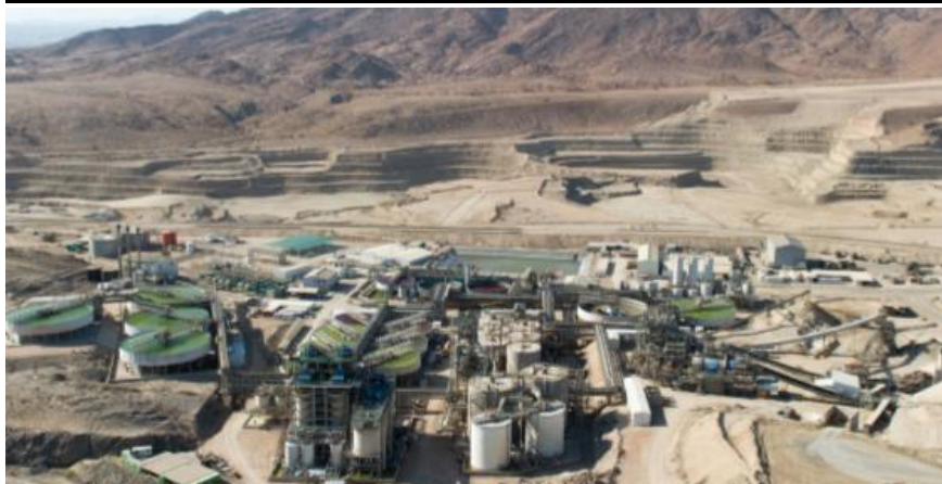
Figure 55: Langer Heinrich Processing Plant
