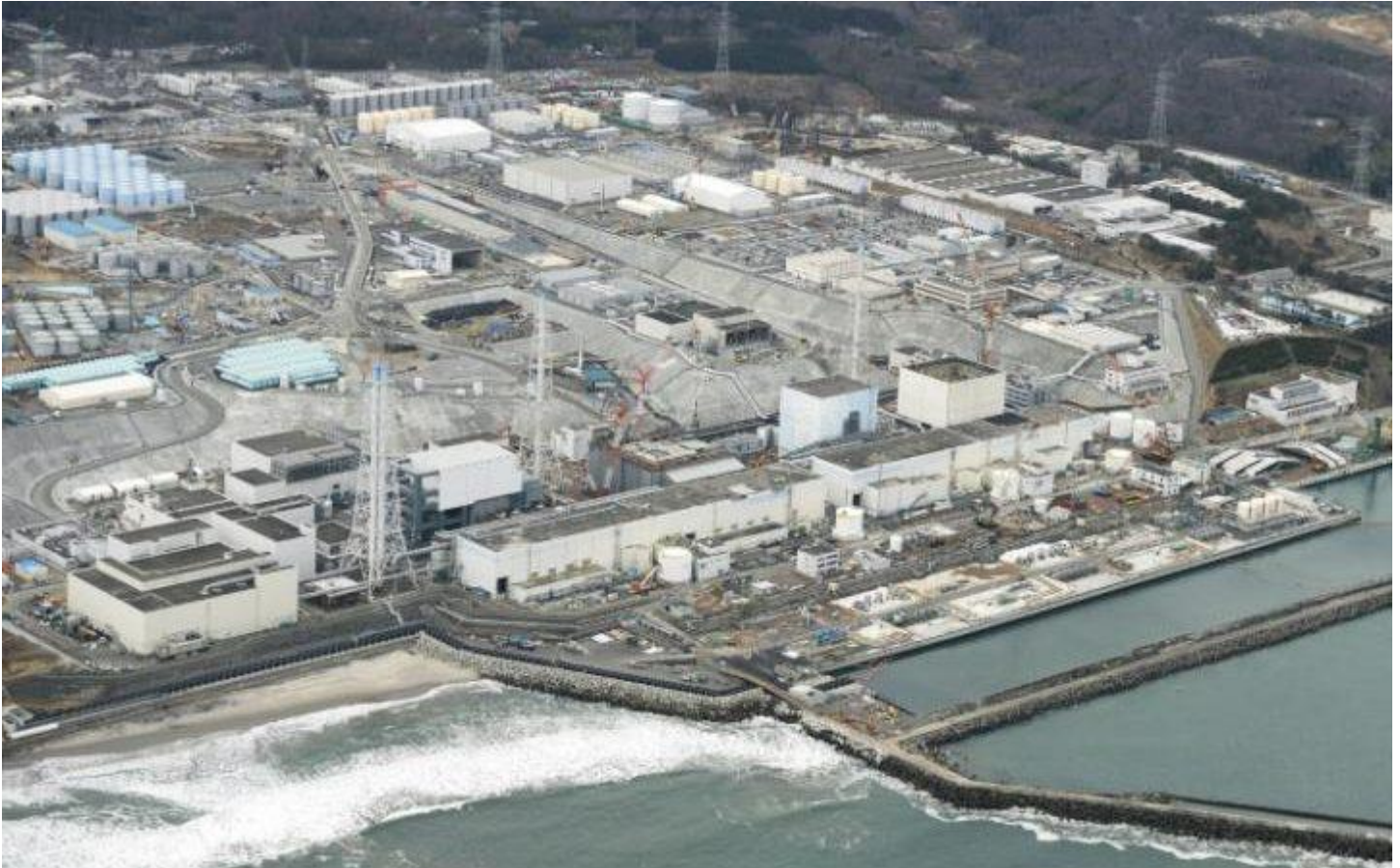
Pictures of the Fukushima plant following the tsunami in 2011
