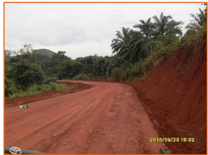
Figure 85: The road to site upgraded
