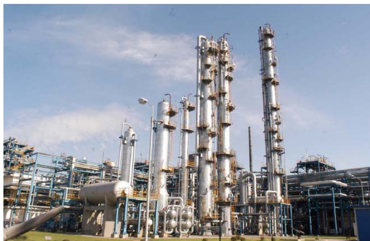
Figure 25: Rectisol Wash Unit by Linde at Jilin, China
