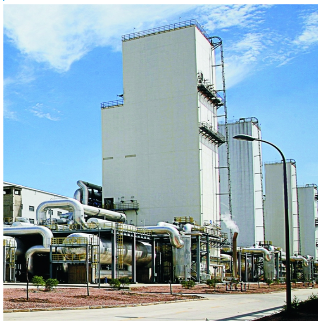
Figure 34: A.S.U. for Shenhua Baotou (2,100 mcf/hr x 4)
