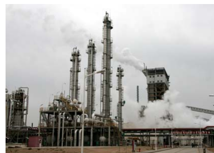
Figure 60: Methanol distillation column in Shenhua Ningxia project
